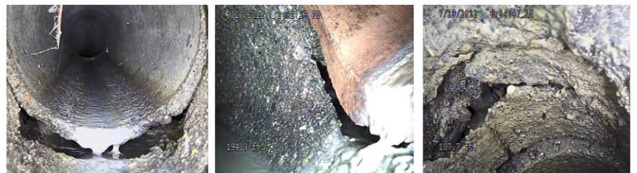
Offset Pipes, Failed Joints, Root Intrusion, Failed Pipes
