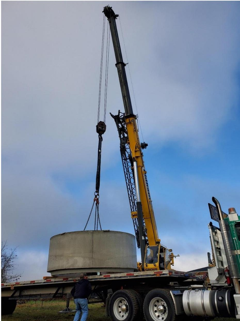
**New Snow Sewer Lift Station Wet Well Section**
