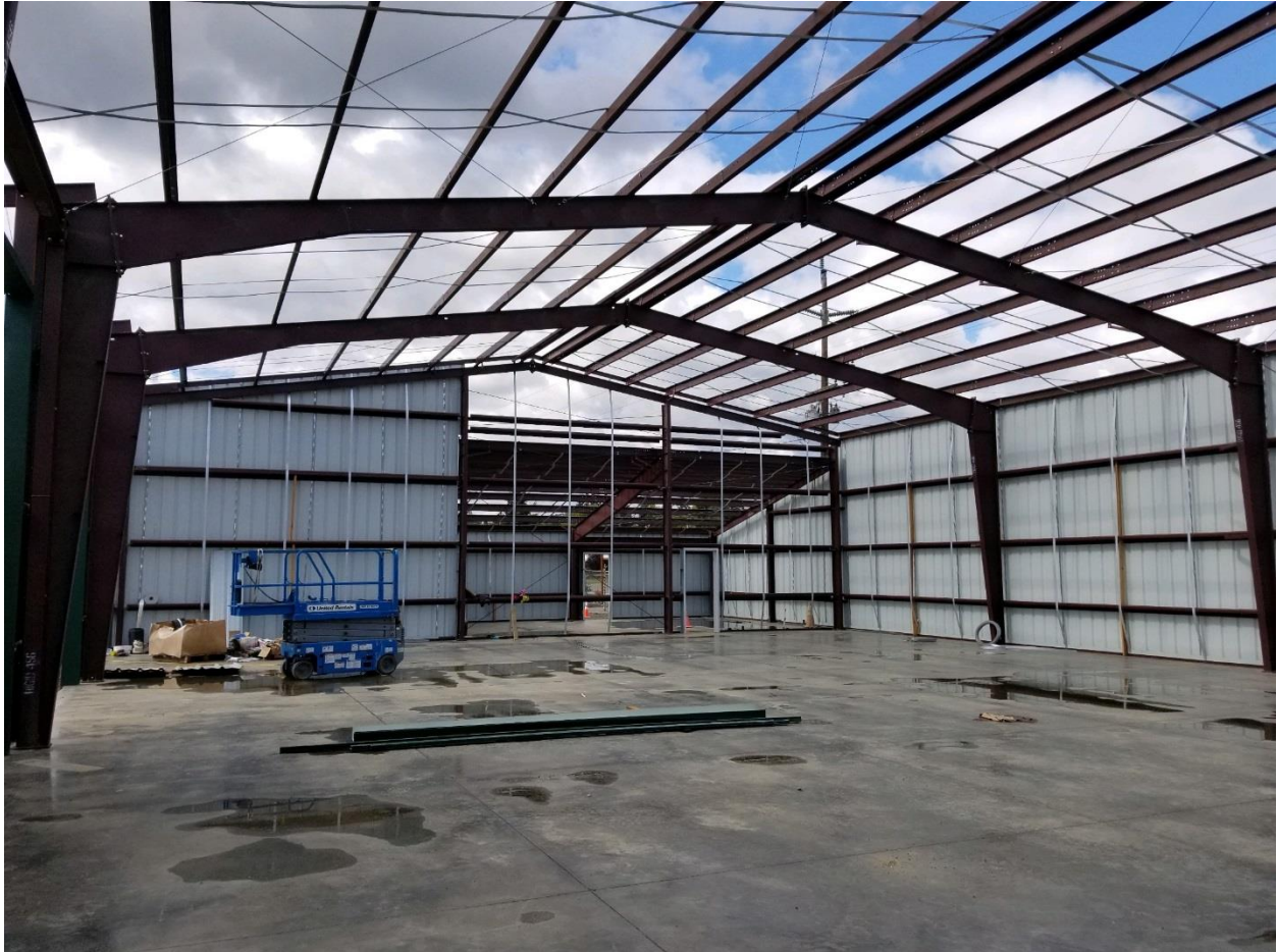
Interior of New City Shop
